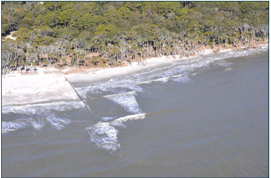
An aerial of a groin on Hunting Island shows the downdrift erosion groins cause
