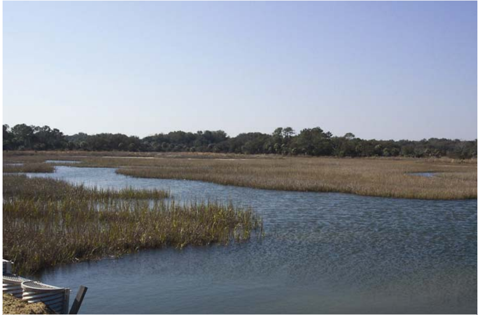
Fenwick Island — this pristine area is where standpipes and fill dirt were installed in the critical area restricting tidal flow to the creek and marsh beyond.
