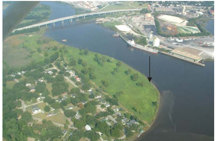
Riverside: the arrow above depicts the area where a developer wants to dredge critical area salt marsh to create a marina basin.
