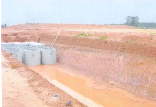
Chem-Nuclear: an unlined burial trench at Chem-Nuclear's radioactive waste landfill.
